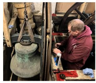
found. (In progress in the picture). The 'set' of the bells has been corrected where necessary and minor adjustments to the fall of the ropes was carried out. Our bells are popular to many ringing teams, and this essential work will ensure their continuance for many years.
